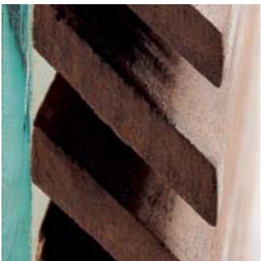
035 Bathroom doors have wooden louvres with glass panels that let in light without compromising privacy.
