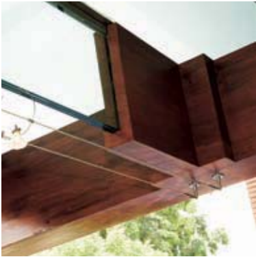
025 The glass deck on the upper level is supported on extra strong PVB laminated glass structural beams. The floor panels themselves can take a load of upto 1.5 tonnes.
