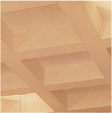
028 The use of coffer slabs eliminate the need for conventional beams and result in dramatically enlarged spaces.
