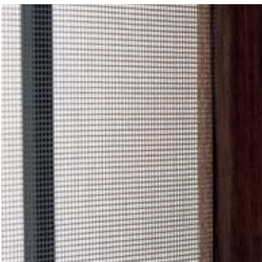
033 Windows and French windows have sliding wooden panels with fine nylon screens to provide protection from mosquitoes and insects.
