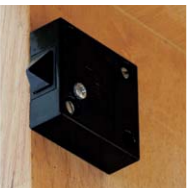
042 Ingeniously placed switches inside wardrobes automatically turn lights on when the door is opened and off when closed.
