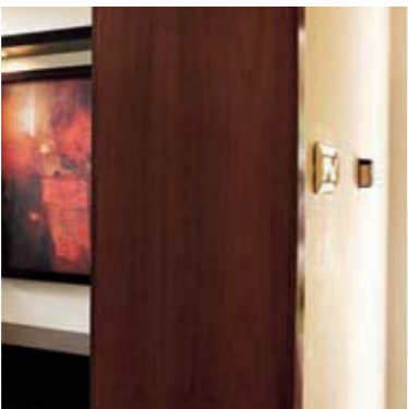
034 Conventional recessed door frames have been replaced by elegant full-width frames that occupy the entire thickness of the wall.
